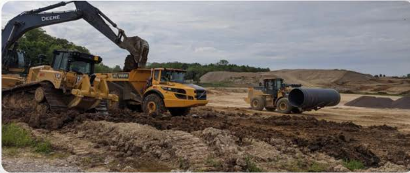
Earthwork | Site Development
